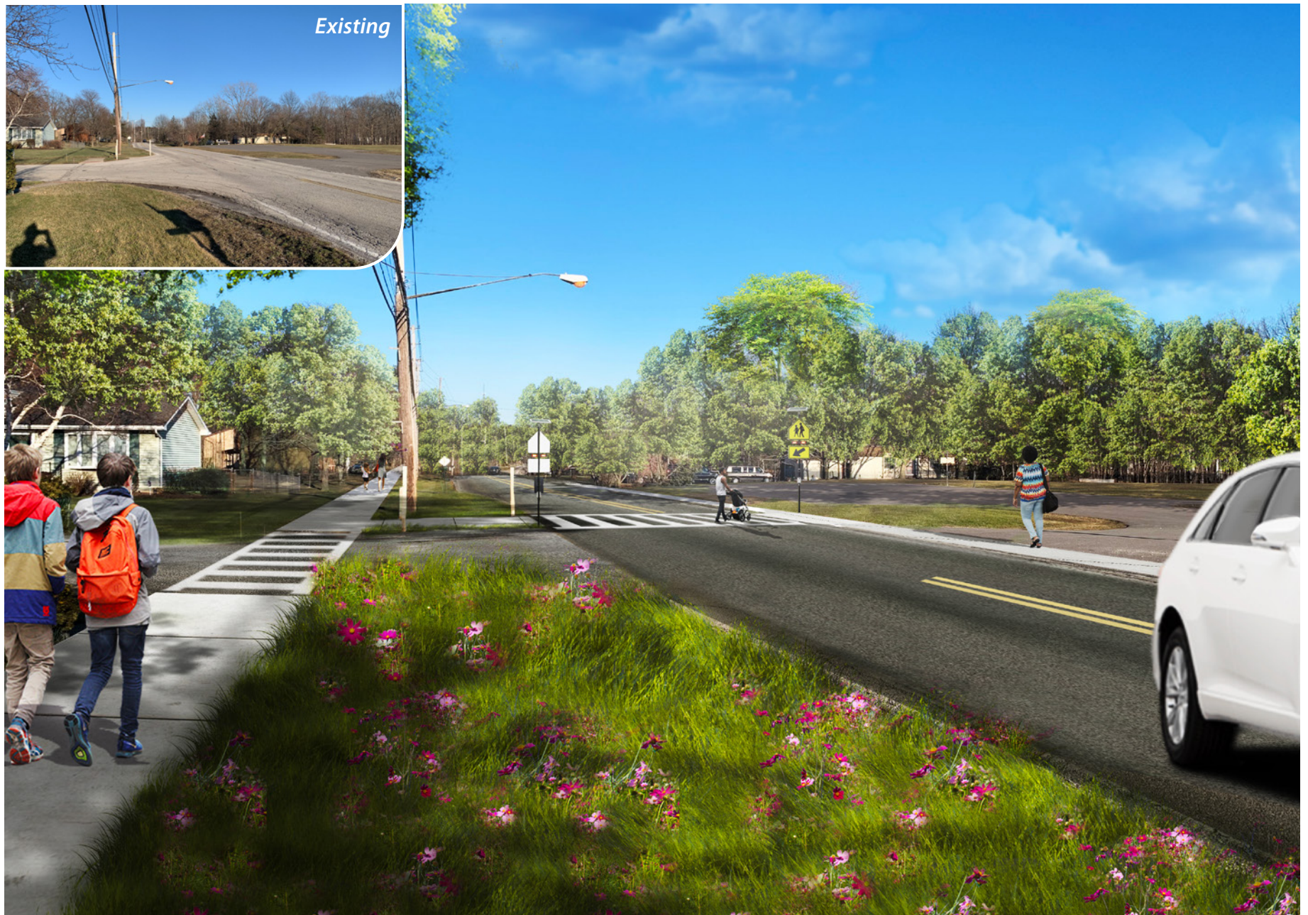
Figure 5. Visualization of Burns Road and Naples Road intersection improvements, including crosswalks, a sidewalk along Burns Road, and Rectangular Rapid Flashing Beacon (RRFB). This preliminary concept is for planning purposes only. Field verification, site condition assessments, engineering analysis, and design are necessary prior to implementing recommendations contained herein.
